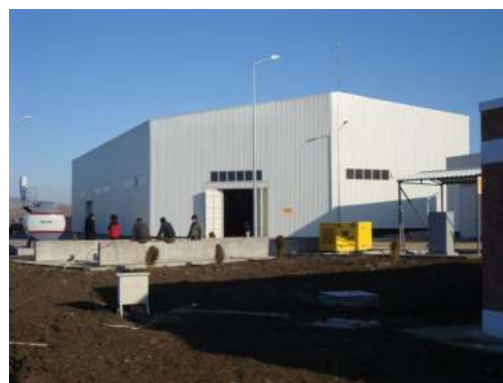
Waste Sorting Building
