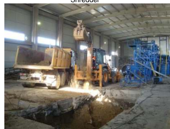
Re-construction of WSL
